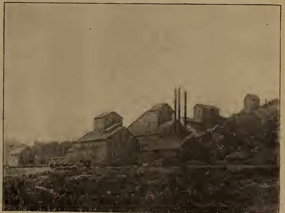
MILL, FROM THE NORTH-EAST.
